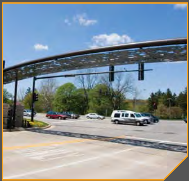
National Metal cut the leafy pattern in the overhead canopy for the entrance of the Morton Arboretum out of 1/2" plate.
